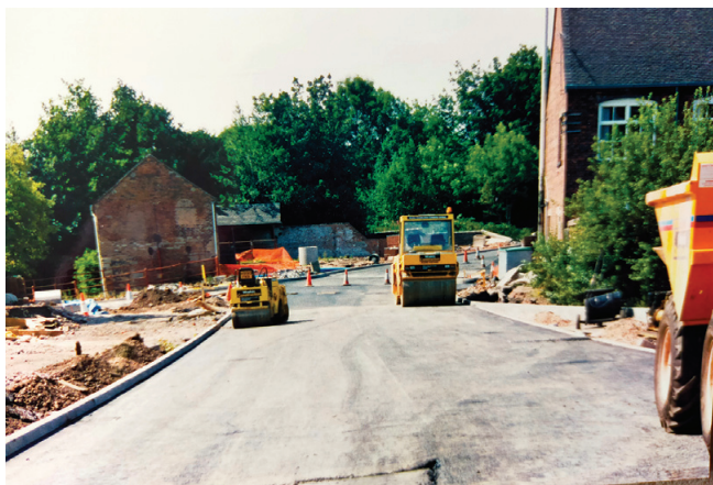
• Construction of Christchurch Way
