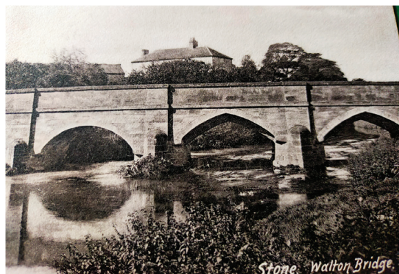
• The old Walton Bridge the two ribbed arches of the original bridge on the right
